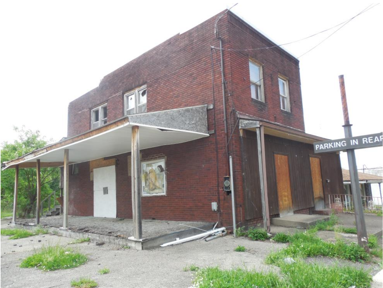
A vacant, blighted structure at 2316 South Ave. has a detrimental effect on the nearby properties and the appearance of the corridor as a whole.
