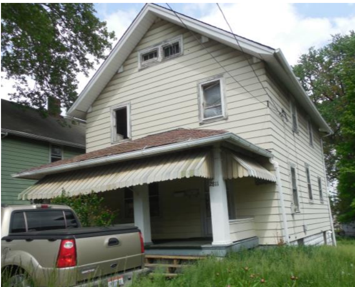
2811 South Ave: DEMOLITION
