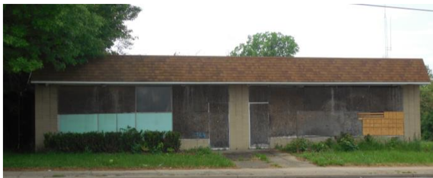
2724 South Ave: DEMOLITION
